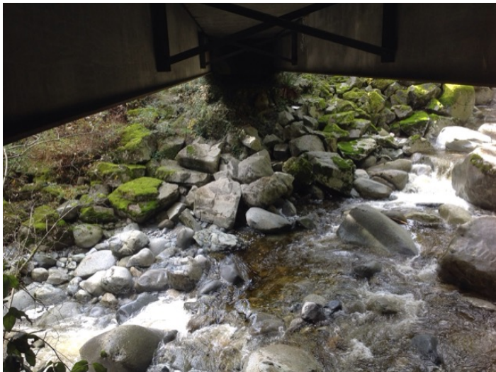
Right Bank Abutment when facing downstream
