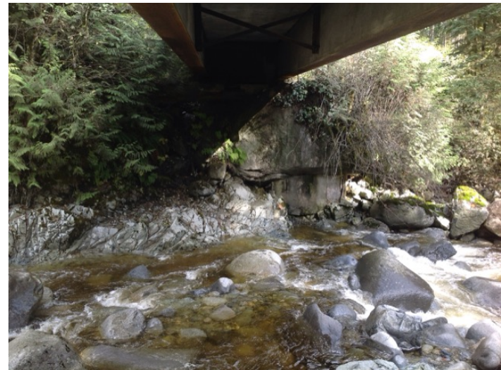
Left Bank Abutment when facing downstream
