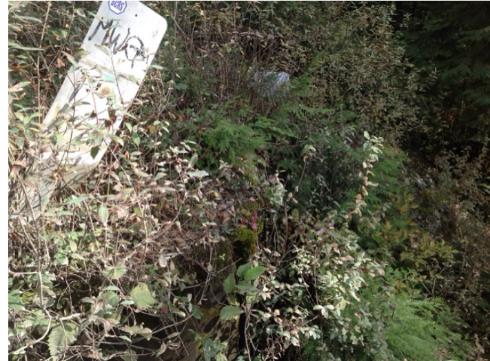
left downstream wing wall
