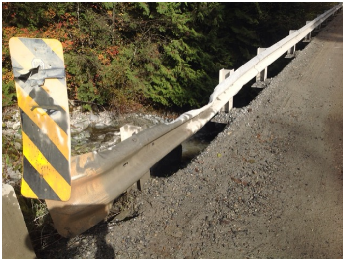
guardrail damage
